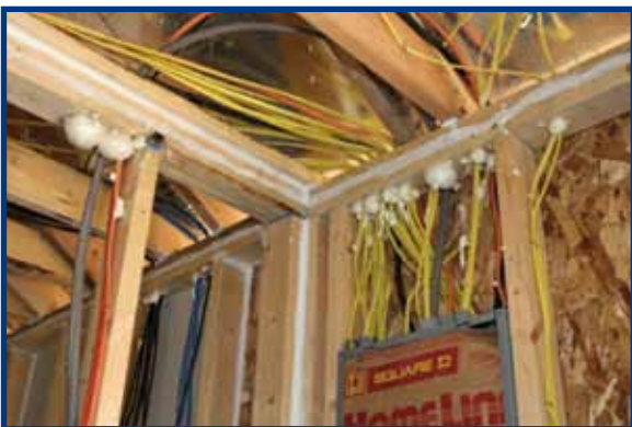
Caulking and Sealing of Top and Bottom Plates, and Electrical Penetrations
