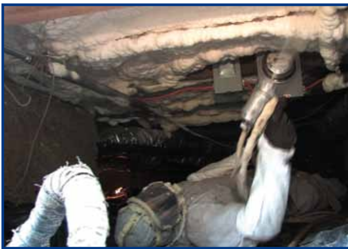
Expanding Foam Insulation Sprayed on Floors
