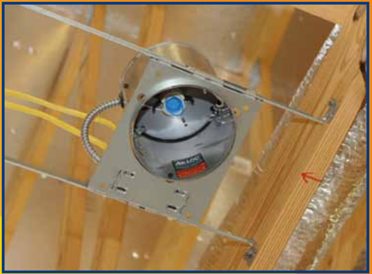
ICAT Recessed Lighting
