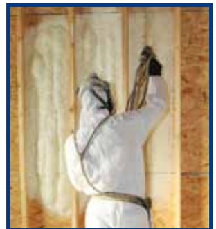
Expanding Foam Insulation
