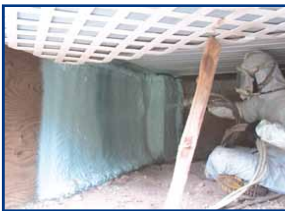
Closed Cell Foam Insulation Sprayed on Crawl Space and Perimeter Walls
