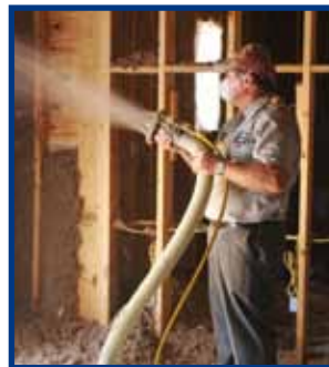
Damp-Blown Cellulose Insulation
