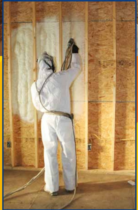
Foam Wall Insulation
