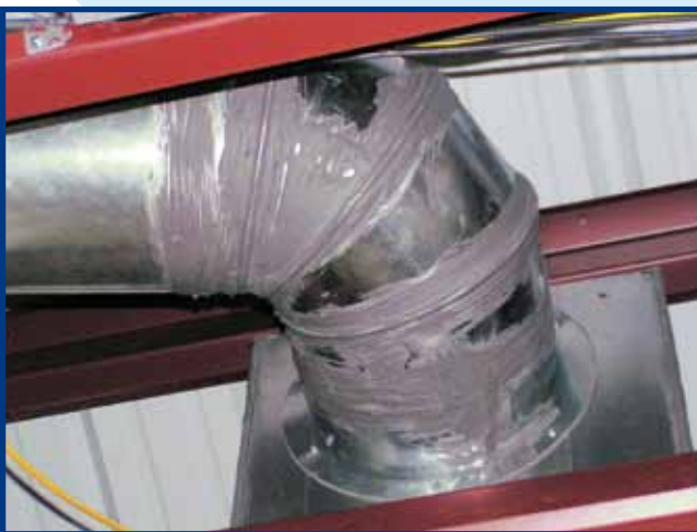
Mastic Sealed Metal Duct
