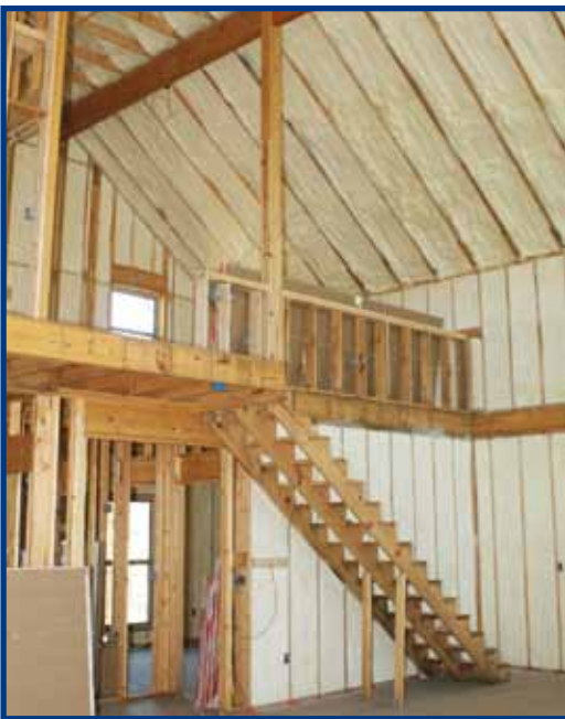
Complete Fill or Cathedralized Foam Insulation
