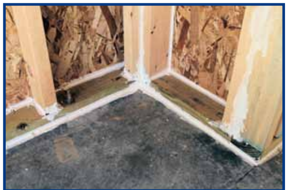
Caulking and Sealing of Top and Bottom Plates, and Electrical Penetrations
