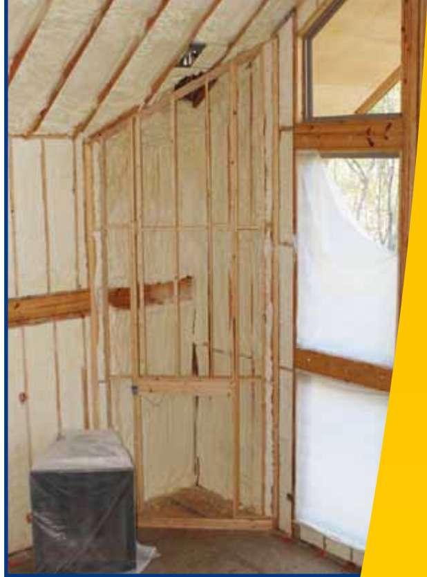
Corner Fireplace Framing Within Foam Insulated Envelope
