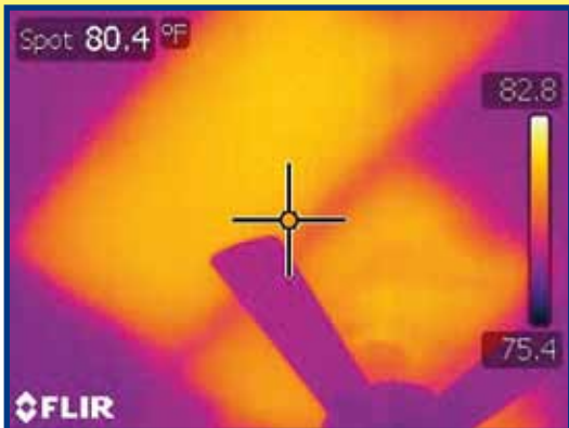
Missing Fiberglass Insulation in Attic
